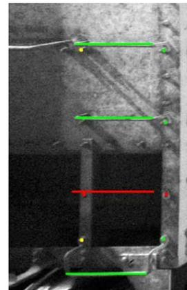
**Figure 6. Missing Ladder Tread**
