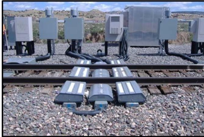
**Figure 11. The Automated Car Undercarriage Inspection System installed on a US Railway**
